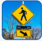
Rectangular Rapid Flashing Beacons (RRFB)
