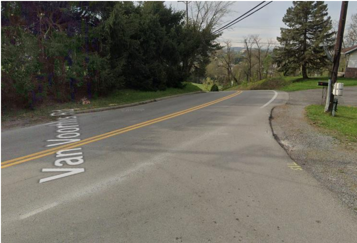
Figure 37: Sight Distance Concerns from Wedgewood Drive Approach
